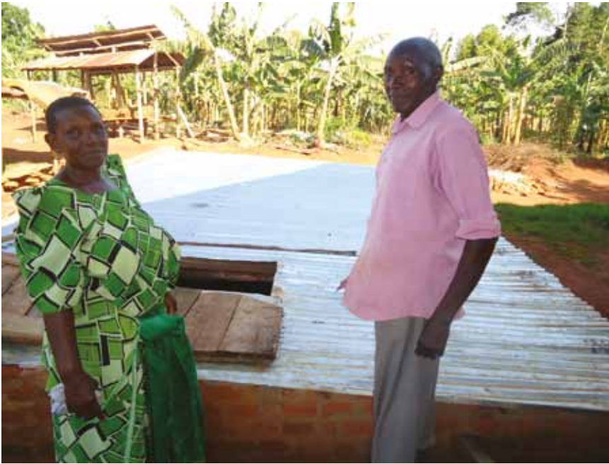
Rain water harvesting tank at the Ddakis' farm
