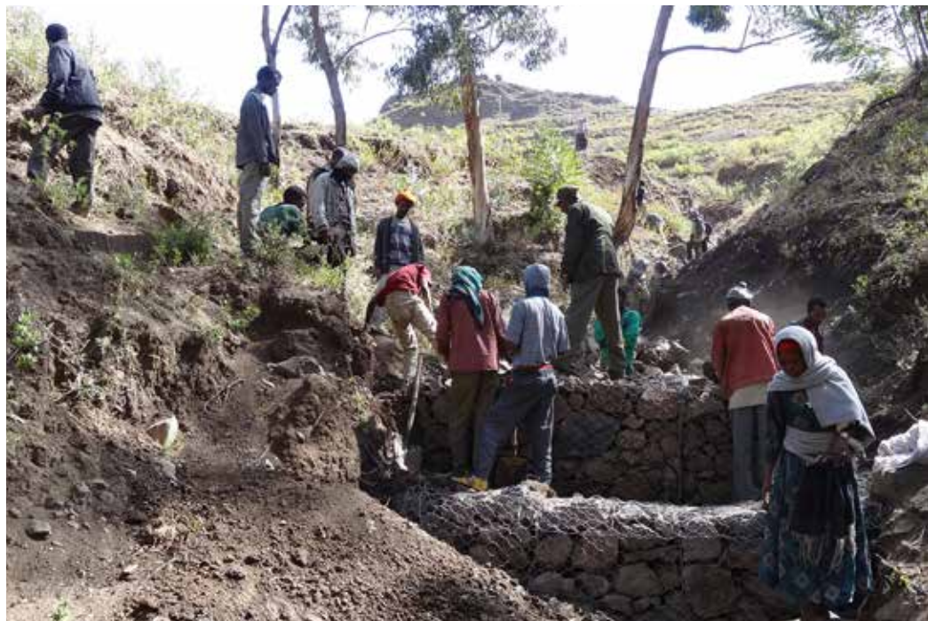
Communities construct gabion check-dams in Zata, Tigray, Ethiopia.
