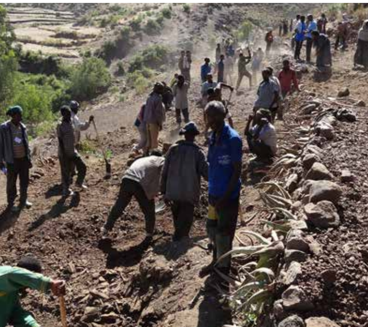
Communities construct bench terraces and deep trenches in Zata watershed, Tigray region, Ethiopia.
