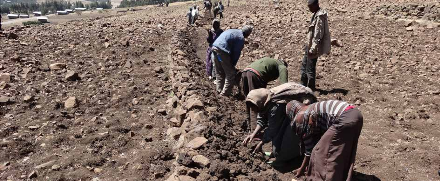
Communities construct bench terraces in Buso watershed, Amhara region, Ethiopia
