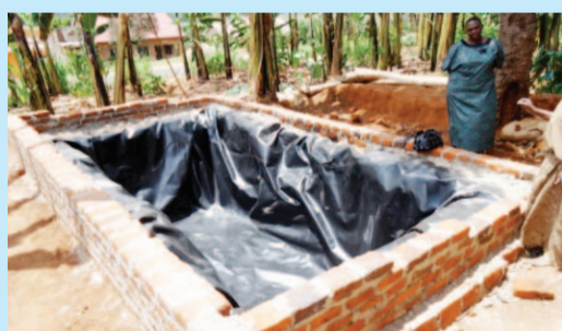
(3) A perimeter wall is build around the pit
