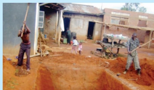
(1) Construction of a pit (6x3.5x2m)
