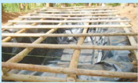
(4) Timber and iron sheets used to cover the tank
