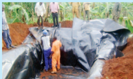
(2) A dam liner saves on cost of sand, bricks and cement used to build the pit
